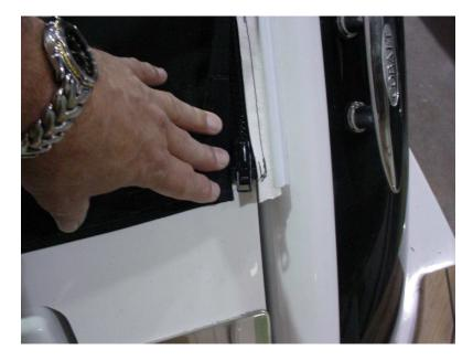
13. Caulk seam between arch and track with silicone caulk. Run a very thin bead, wet with soapy water, and smooth with finger.
