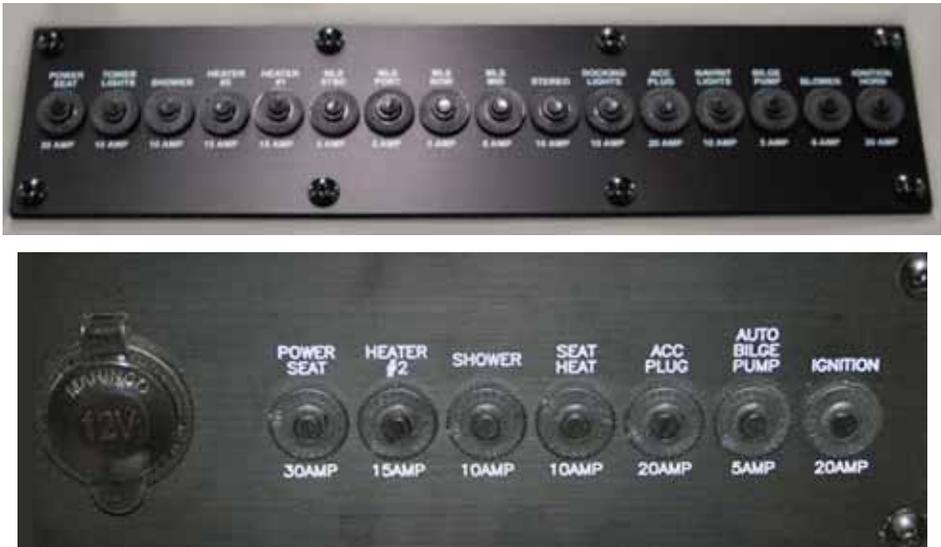
Figure 2-13. Circuit Breaker Panels
