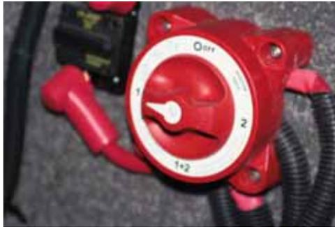
**Figure 4-10. Battery Switch**
